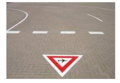
n) Holding Point: Runway holding point markings on taxiways identify the location where an aircraft/vehicle is required to stop when it does not have a clearance to proceed onto a runway.
