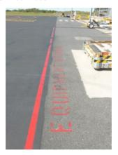
c) Equipment clearance Lines are identified by a broken red line. They define areas where vehicles and equipment may park in the short-term, awaiting the arrival of an aircraft. Vehicles and equipment must remain behind these lines until the aircraft red anti-collision beacon is extinguished.
